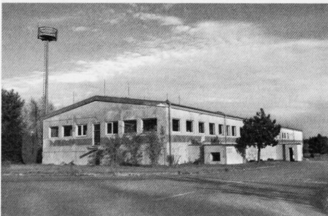
Missile Command Post building, the two porches protect emergency exits from the "bunker".
